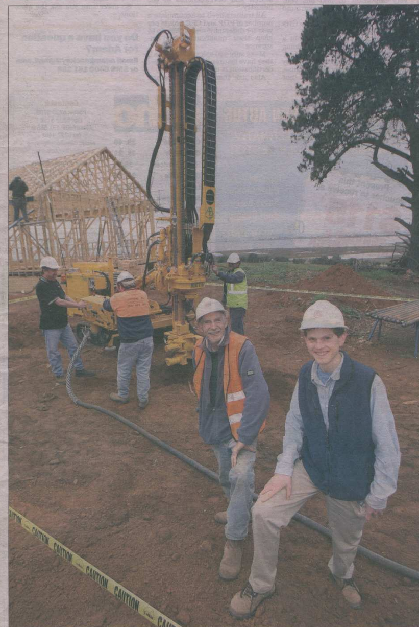
Property owner Ted Payne and son Donald beside the drilling rig.
